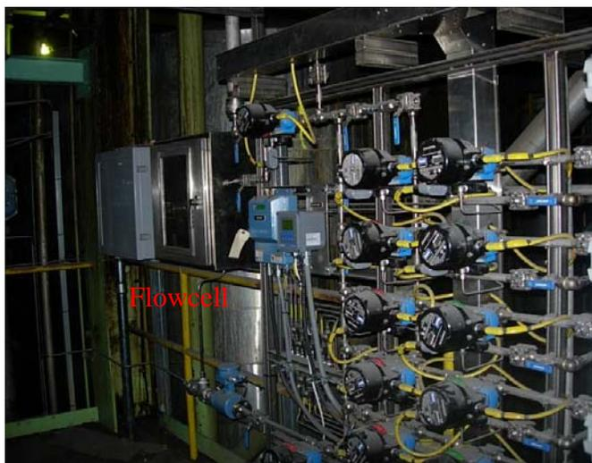
Figure 1B. Actual installation at a Mill, showing valve installations for dissolving tank liquors, equalization tank liquors, and weak wash.
