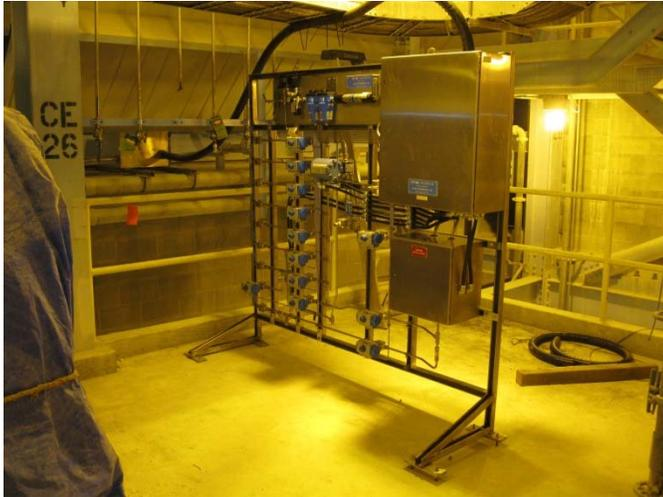
Figure 1: Celgar's FITNIR Analyzer Sampling Skid: six sample streams (RGL, CGL, WW, WL, #1C, #4C), shown without roof and plastic cover.
